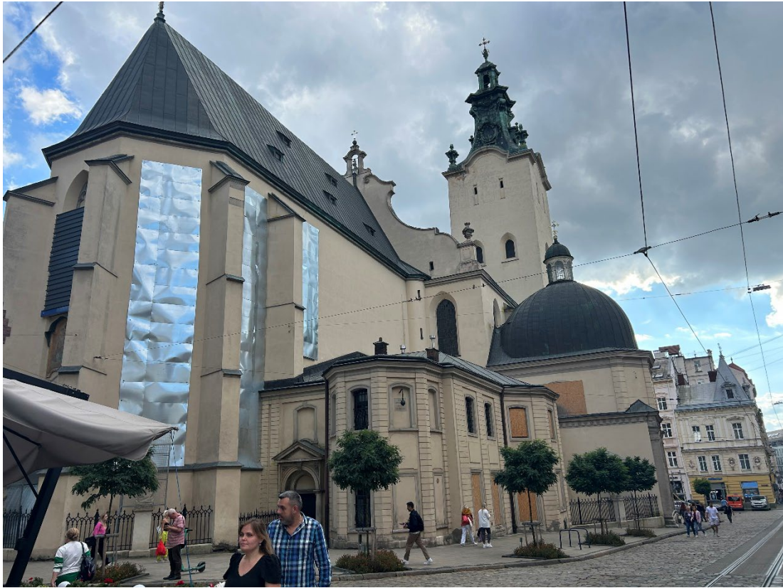
The Catholic Cathedral, windows protected.
